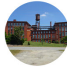
Gentrification in 1995 saw the old Mill turn into Fulton Cotton Mill Lofts
